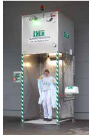
Tanknotduschen Tank safety showers
