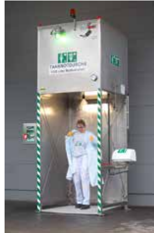
Tanknotduschen Tank safety showers
